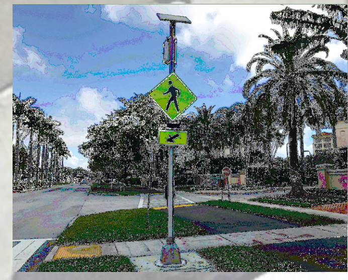
SOLAR POWERED BEACON CROSSING
